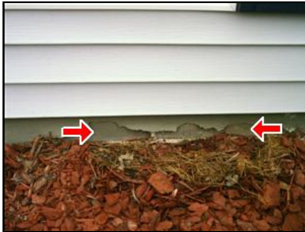
5.0 Picture 1 Water barrier, front of home
