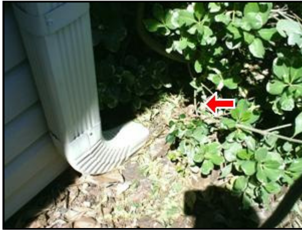
1.3 Picture 1 Downspout left front of home
