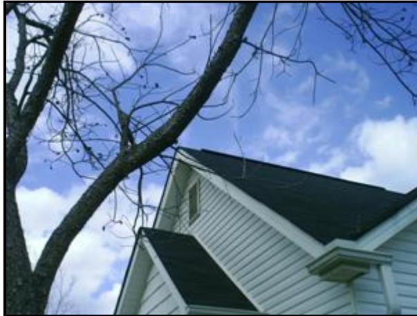
2.4 Picture 1 Limb overhanging roof.
