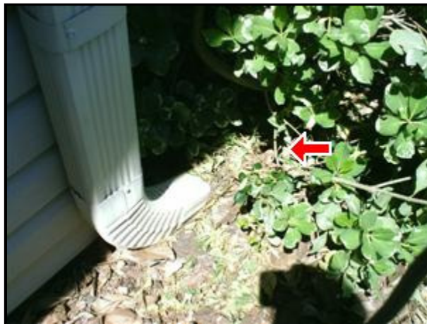
1.3 Picture 1 Downspout left front of home
