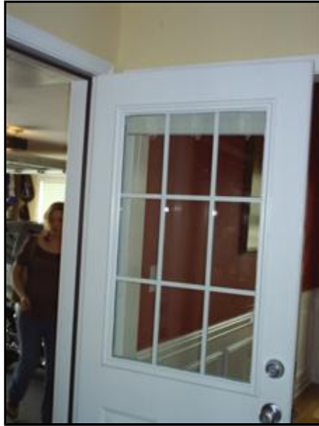
3.4 Picture 1 Garage to dwelling door.
